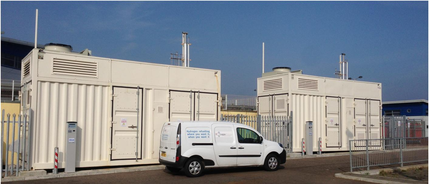
H2Tec's H2Key Gen is a self-contained, fully integrated hydrogen refuelling station for hydrogen vehicles. In its full format it generates hydrogen from local water and electricity supplies, and compresses, stores and dispenses it to provide an autonomous transport refuelling system.
